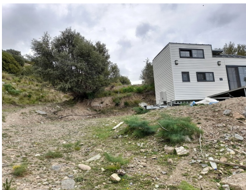
First accommodation unit during construction.
